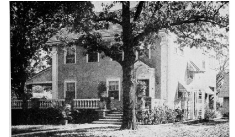
Residence of Mr. E. R. Mason, Des Moines, Iowa. Architect, C. E. Cope. Stucco on Sykes Expanded Cup Metal Lath.
