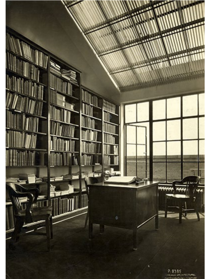
The NAR Library as it looked in the 1930s, in the 59 E Van Buren building
